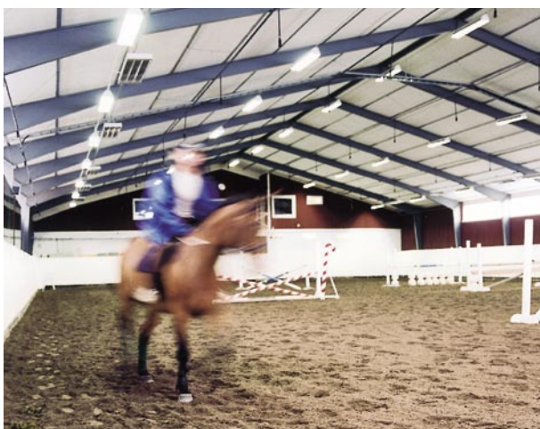
Radiant heating heats people directly without warming the surrounding air. The operative temperature, i.e. the temperature a person senses, is therefore a little higher than the actual temperature. Every degree reduction will save approximately 5% of the energy consumed!
